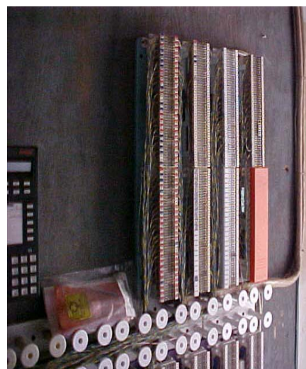
New Telephone Wiring Termination Installation
