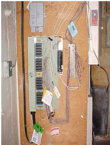
Existing Telephone Wiring Termination Installation
